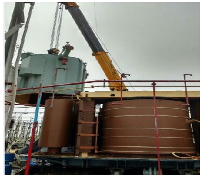
Fig. 11. Inspection of active part of transformer
