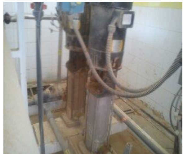
Fig.2.Two high pressure pump motors for (RO system).
