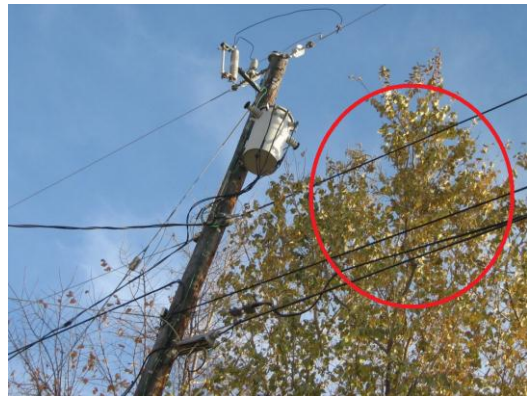
Fig. 1 Connection probability among conductors and foliage.
