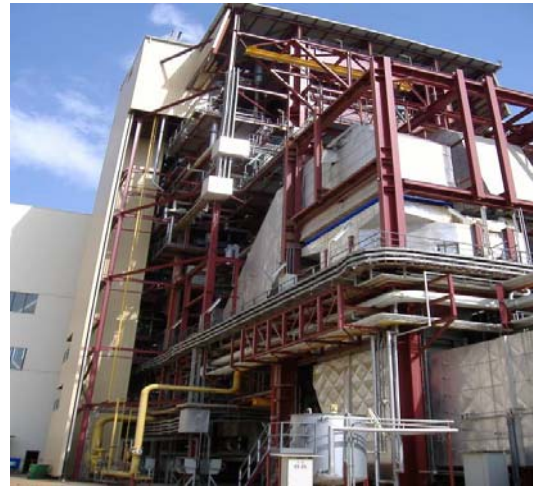
Fig. 3. Example of a boiler of a TPP
