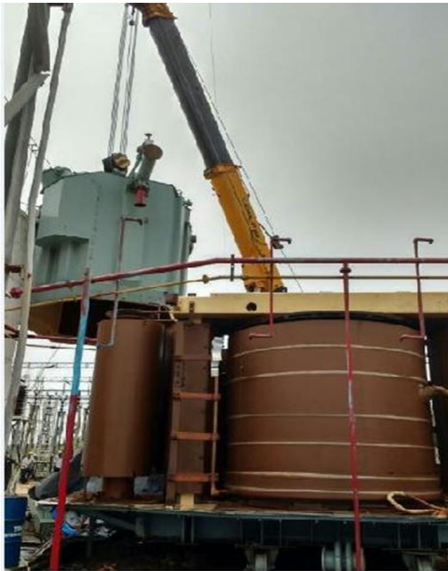
Fig. 3. Inspection of active part of transformer
