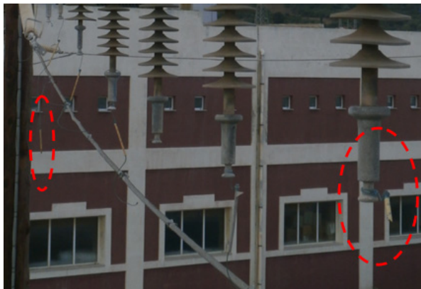
Fig. 6. A close-up photo from 150kV suspension insulators installed in TALOS following the initial scheme. The connecting wire of the far left fuselink has been cut off and the far right fuselinks has shattered.
