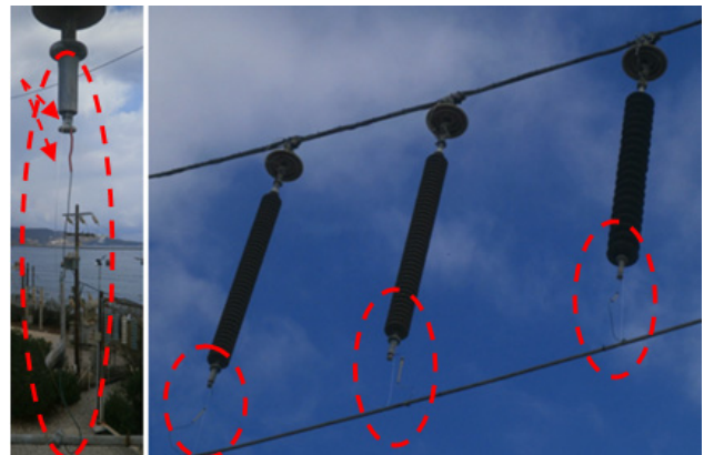
Fig. 7. Close ups from 150kV suspension insulators installed in TALOS with a non-conductive high strength net used to absorb the mechanical stress.
