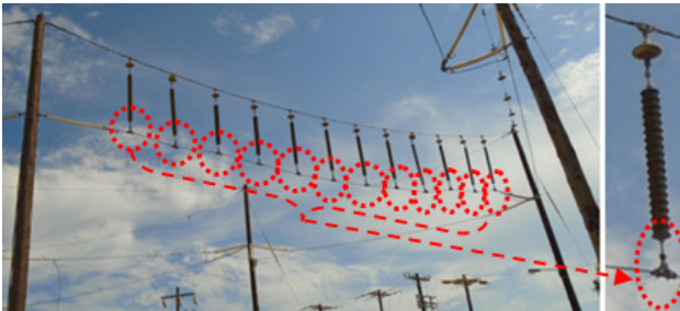
Fig. 10. The final set-up scheme followed in TALOS. The expulsive fuselinks have been fully removed.
