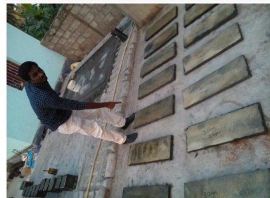
Fig.I. Ferro cement slabs during and after casting
