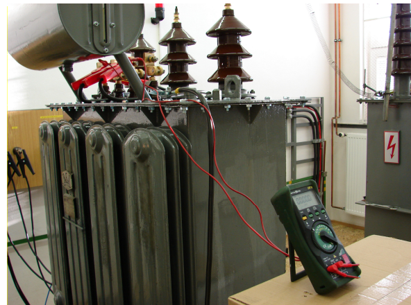
Fig. 1. Measured transformer 630 kVA, 22/0,4 kV, 16,5/909 A after disconnection from operation
